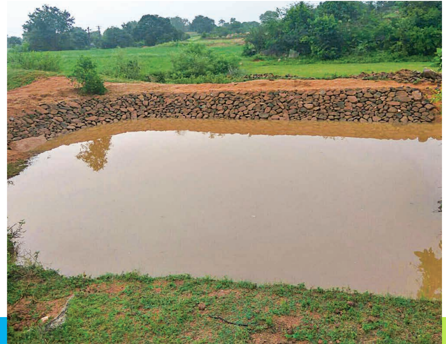
Dugout pond built by villagers as part of watershed programme in Siddipet in Telangana, India
