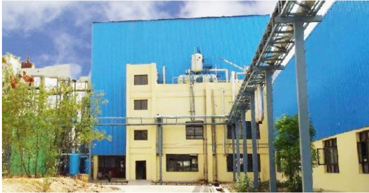
At Malanpur, we installed a 14 tph capacity biomass boiler to help us replace fossil fuel and utilise renewable energy resources
