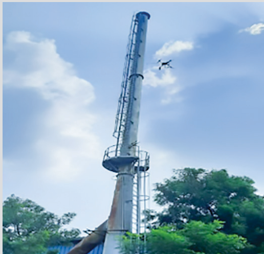
Using drones for smoke stack inspection at our industrial chimneys
